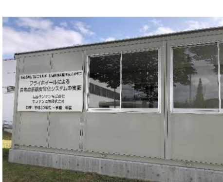
(a) control room
